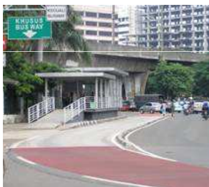
Figur 3.26 BRT-station i Jakarta
